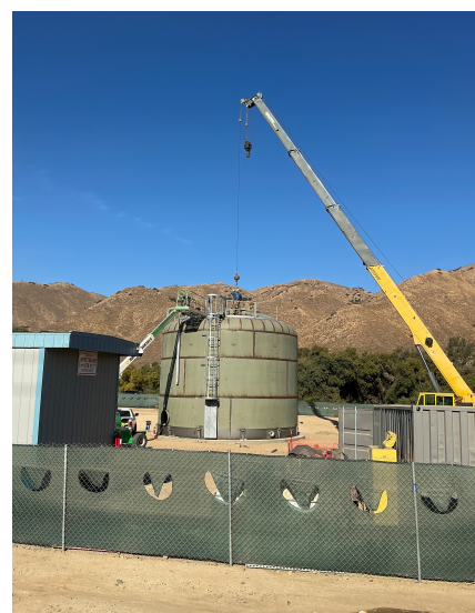
Steel Tank Construction
