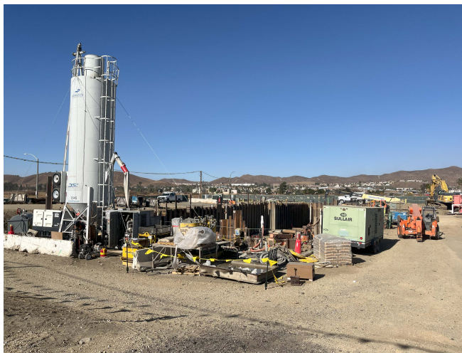
Sewer Lift Station Shoring
