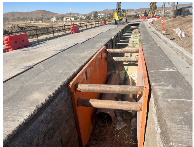
Dual Force Mains Construction
