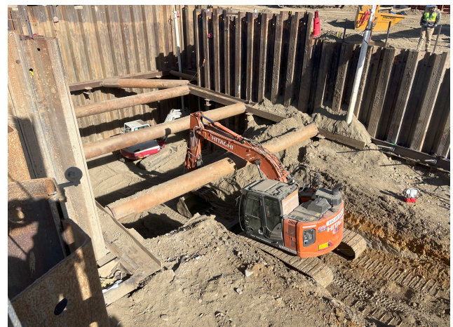
Sewer Lift Station Excavation
