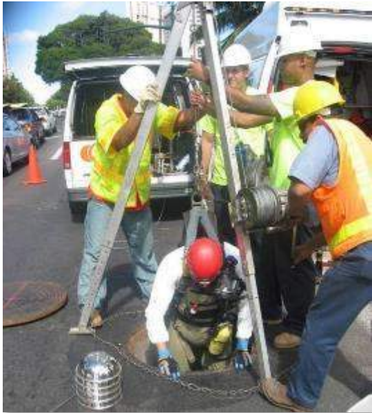
Photo 2-1. Confined Space Entry
