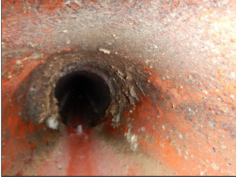
W Influent Pipe
