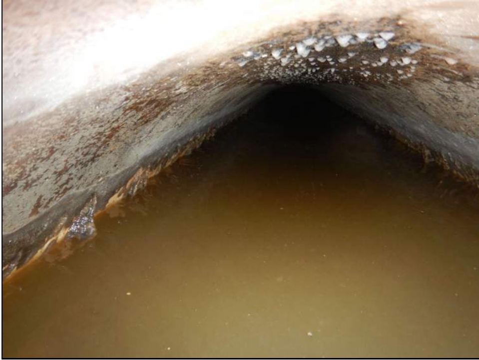
Monitored SE Influent Pipe
