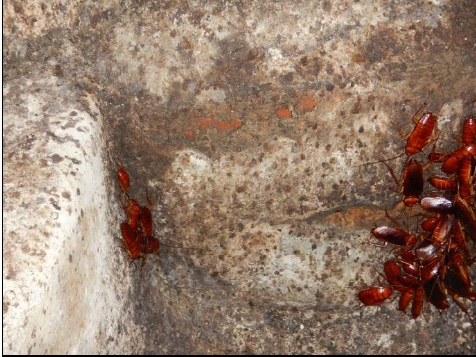
W Influent Pipe
