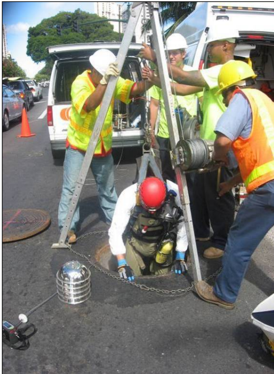
Photo 1. Confined Space Entry
