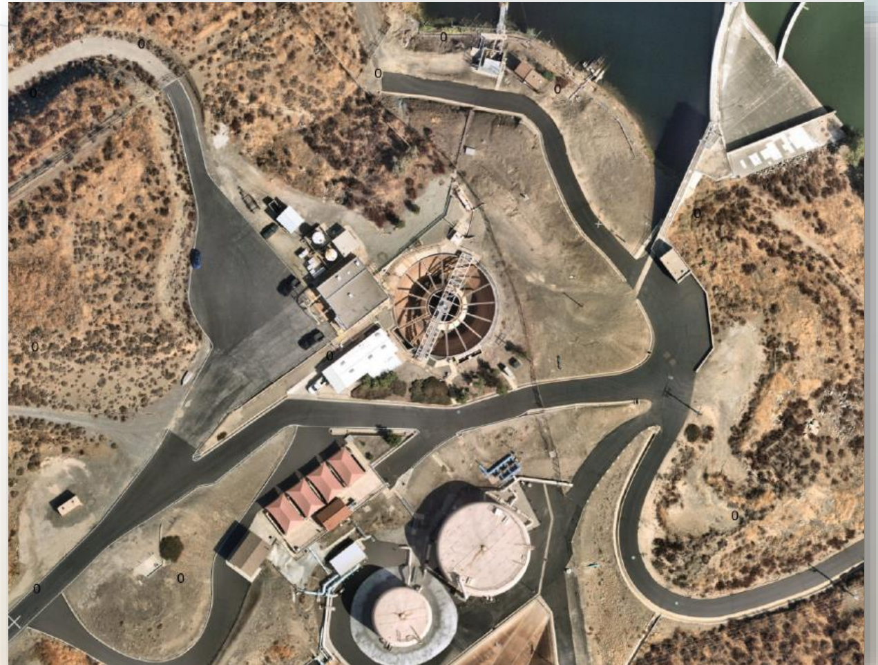
Aerial image of the treatment plant
