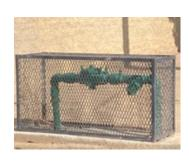
Enclose the backflow preventer within a protective cage. The cage should be secured or mounted to the ground.
