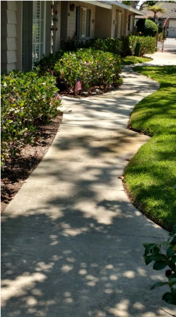
When this community was originally built the soil was below the grade of the structures. No longer. In a heavy rain this bugling landscape will shed water instead of absorbing it, endangering the homes, walkways and public safety.
