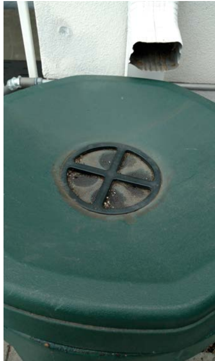
Not only will this fine-mesh screen prevent debris from getting into the rain barrel, but also mosquitos.
